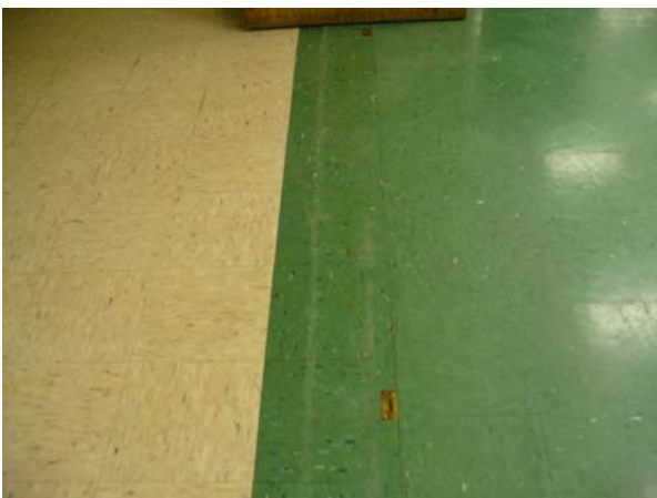
Broken VCT at Cafeteria
