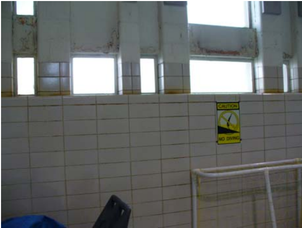
Deteriorating Window Assembly in Pool
