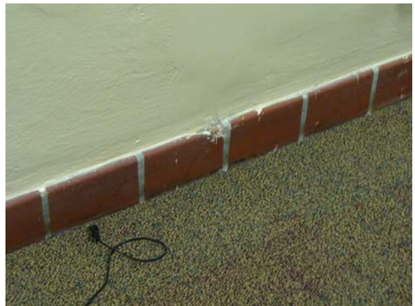
Typical Tile Base Damage
