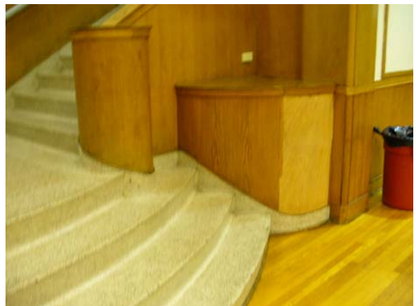
Missing Paneling in Social Room
