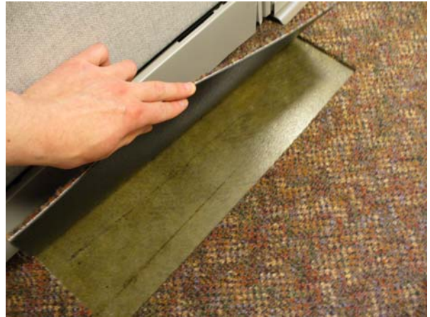
Poorly Adhered Carpet Tile in Offices
