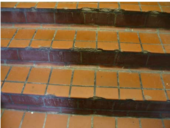
Damaged Tile Stairs
