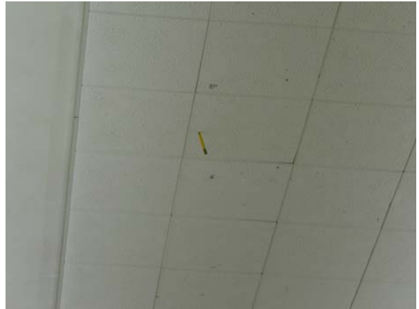
Typical Ceiling Damage
