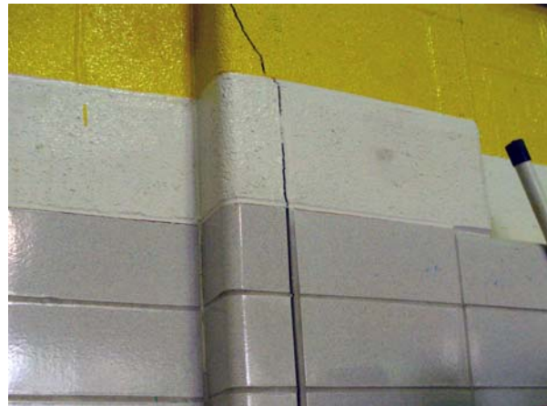
South Pool pilaster
