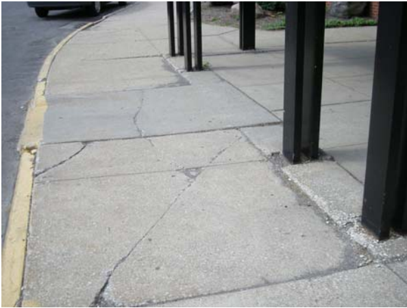
Typical Concrete Walk Damage
