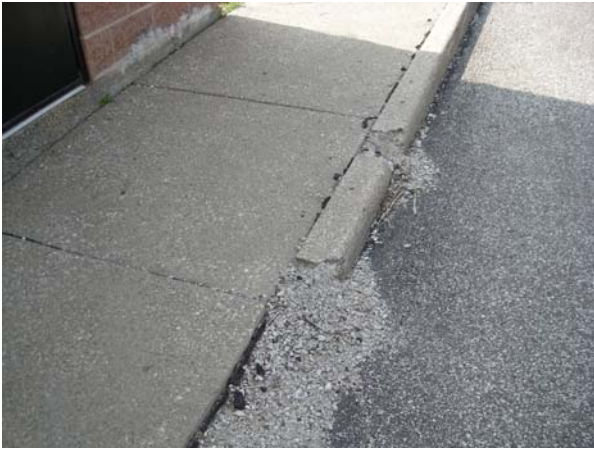
Typical Curb Deterioration
