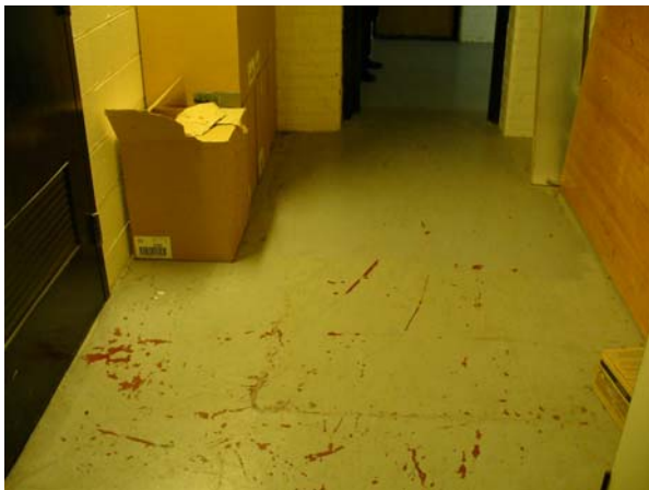
Typical Lower Level Concrete Floor
