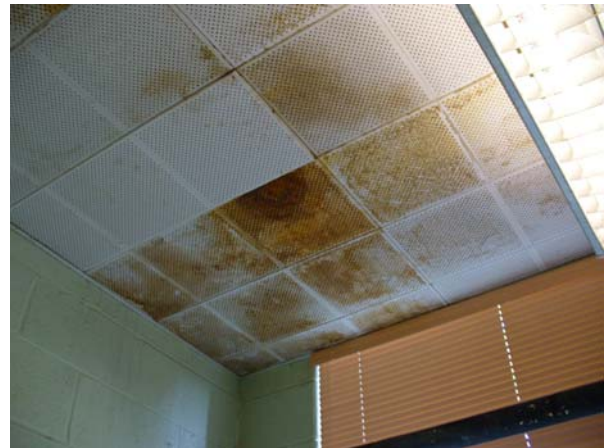
Rusted Metal Ceiling at Science Wing
