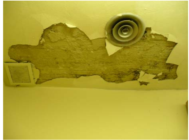
Water Damage at Ceiling
