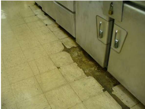
Deteriorating VCT at Kitchen
