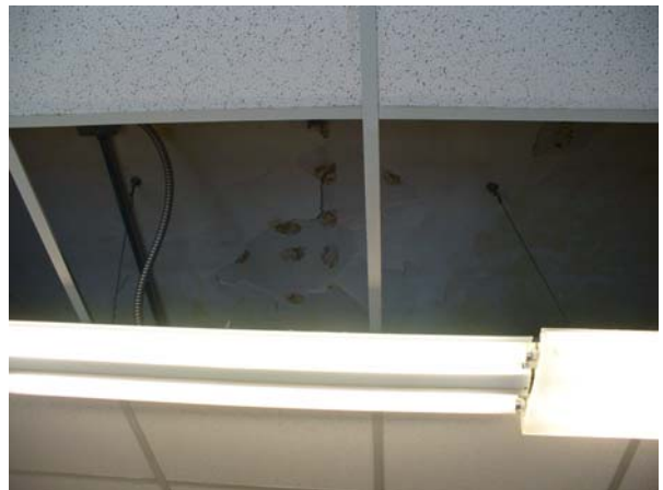
Ceiling in Offices
