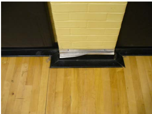
Bent Pad Track in Gymnasium
