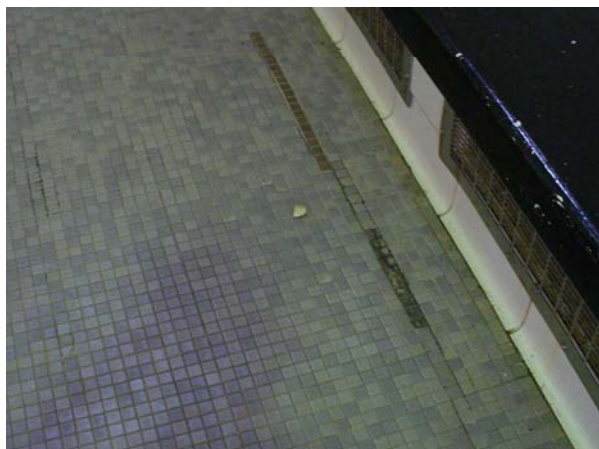
Cracked Tile at Pool
